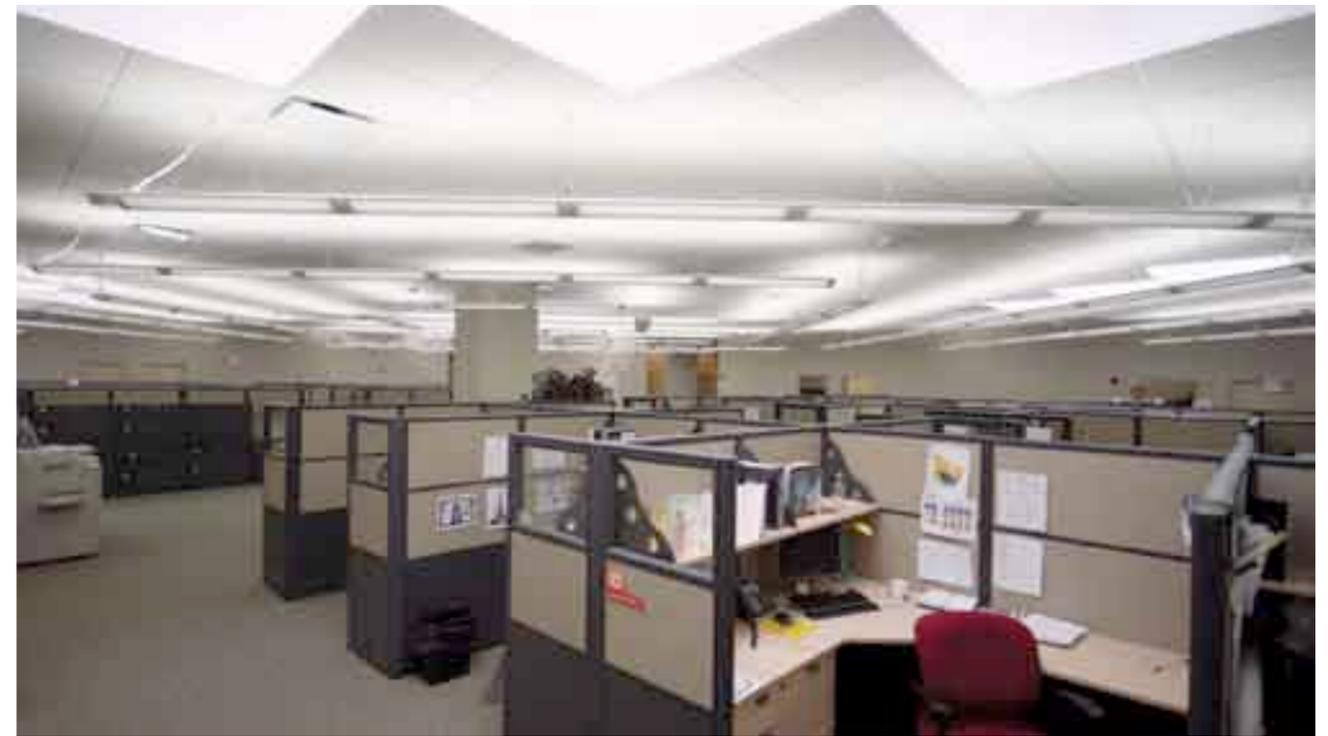
**LIGHT TOUCH** Six daylighting units, incorporated into the ceiling tile, bring diffused natural light into the office area.
