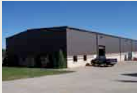
County Fire Protection's New Brimfield Facility
