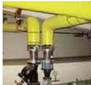
Bay Mechanical's award-winning project at Cleveland State University
