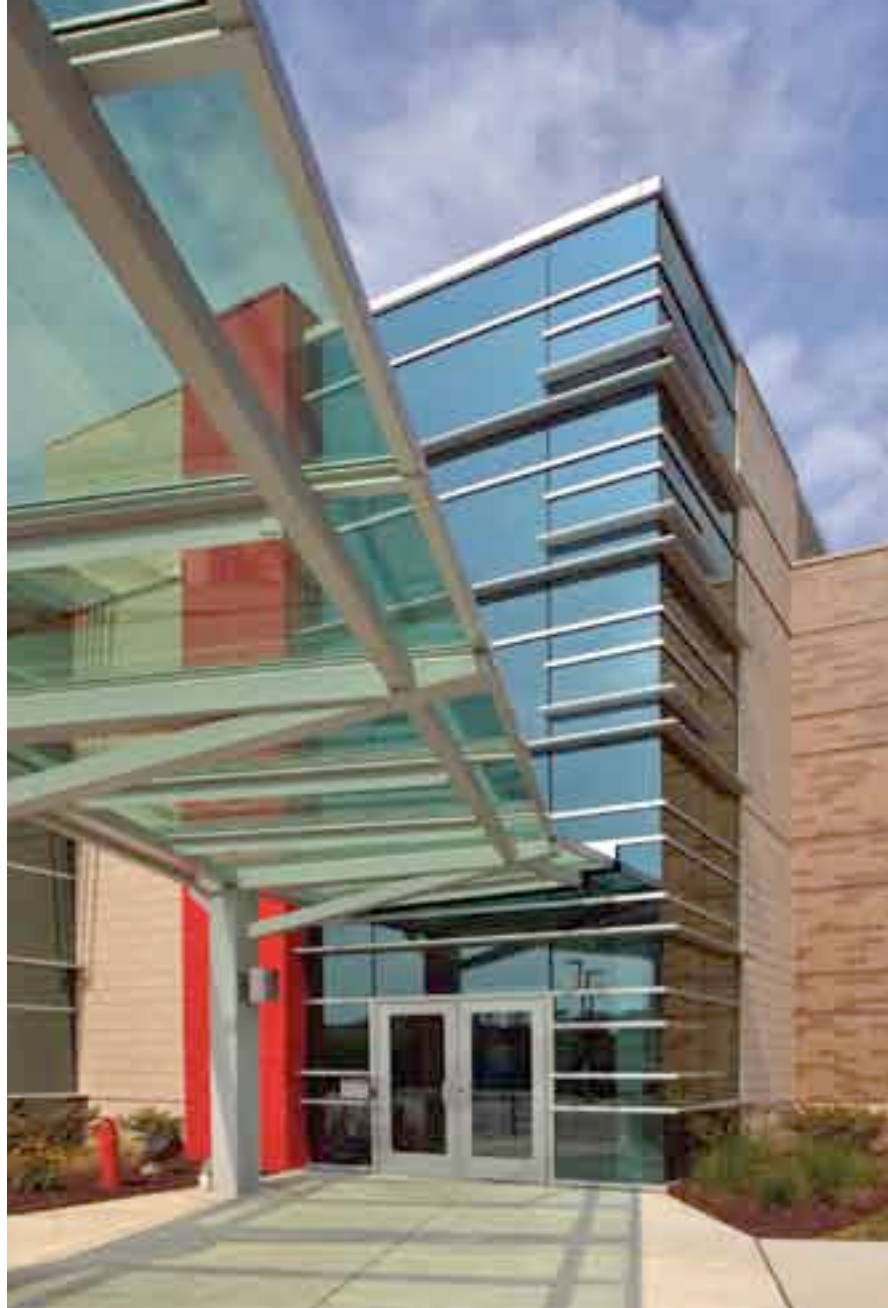
FORWARD FORMS “We were trying not to make it like a typical office building,” says Michael Christ, project architect with Vocon. “We were trying to use some of the more modern materials like the metal panels, and the large expanses of glass.
