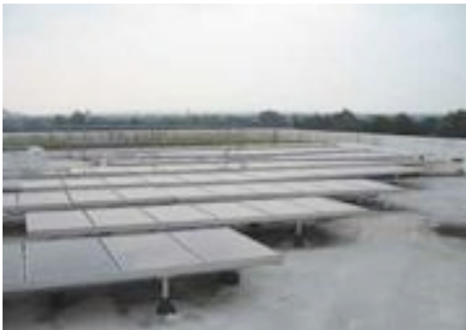
SMART SYSTEMS An early green project in Northeast Ohio was the Cleveland Environmental Center, which opened in 2003 and features a green roof and solar panels.
