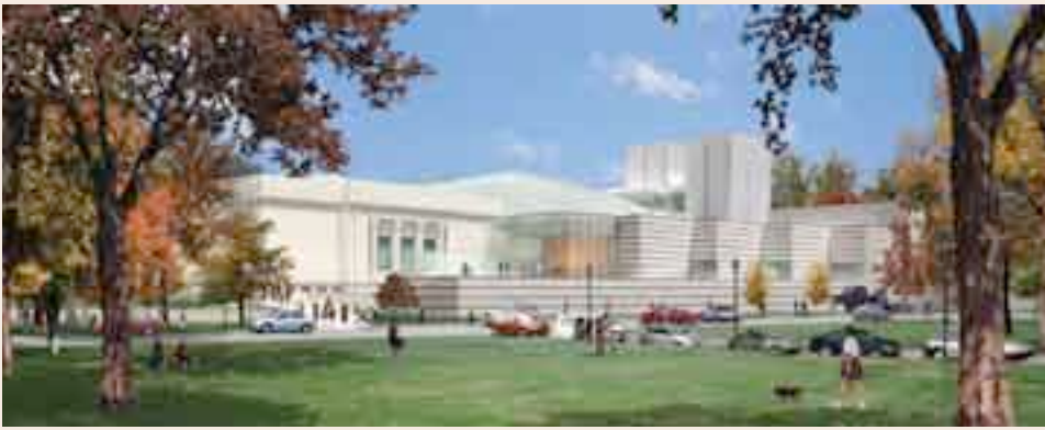
FOCUSED ON THE FUTURE The renovation and expansion is scheduled for completion in 2012.
