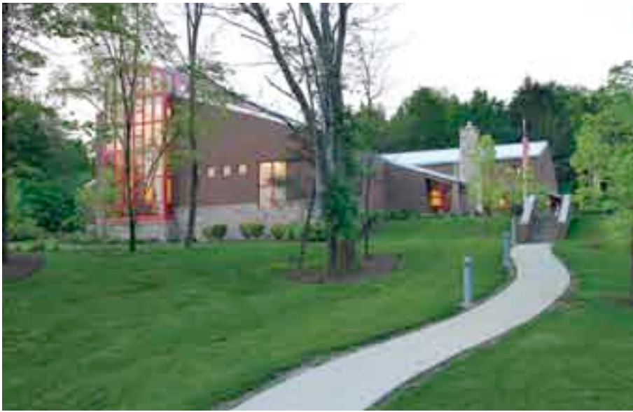
FARM + FUTURE The new Lodi Library is intended “to evoke an image of a barn, but also to stand on its own as a fresh piece of architecture,” says Principal Architect David Milling.
