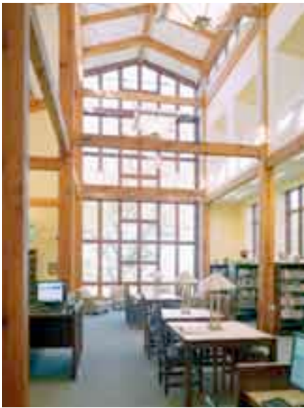
TIMBER TOP Post-and-beam construction provides the new Lodi Library with a warm, open and rustic environment.
