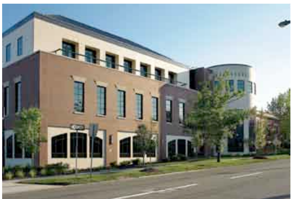
BREAKING DOWN DESIGN Adding a recessed third story and using a mix of materials and colors were techniques employed to decrease the size and mass of the Medina Library addition, according to Architect David Milling.
