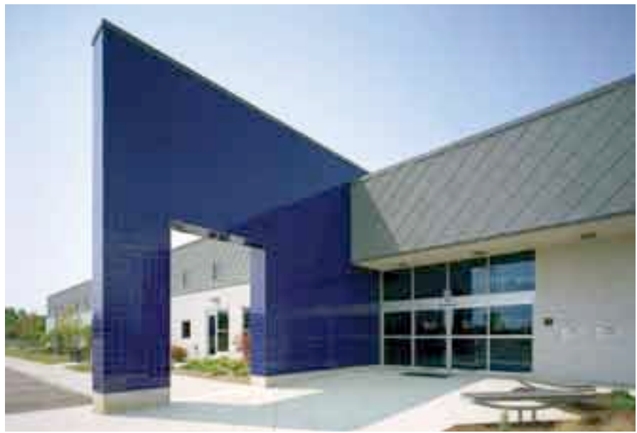
GREAT DIVIDE A massive cobalt blue, tiled wall separates public and back-of-house operations at the new Buckeye Library.
