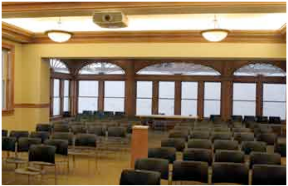
MAKING ROOM To provide a space large enough to accommodate up to 80 union members, several interior walls and support columns were removed on the south end of the mansion.
