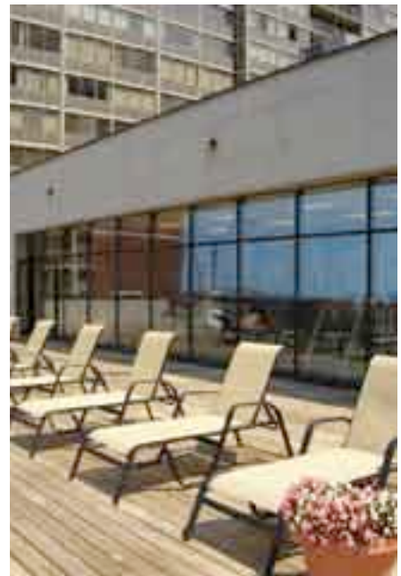
LIGHT TOUCH The renovated Embassy Suites Hotel includes fitness resources, a sun deck and more.
