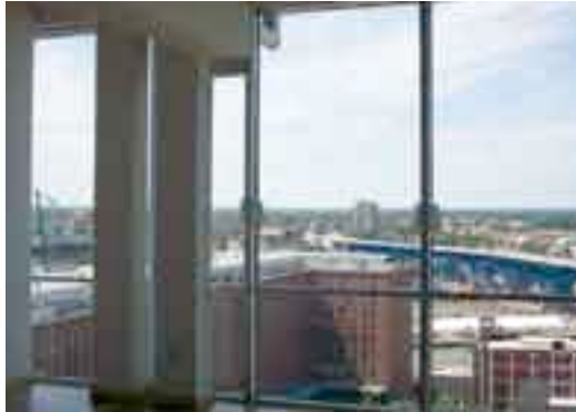
DEGREES OF DIFFERENCE Films vary in weight from the lightest (70 with 17-22% protection) to the heaviest (40 which is the darkest and has 99% UV protection). The lighter the film, the clearer the window.
