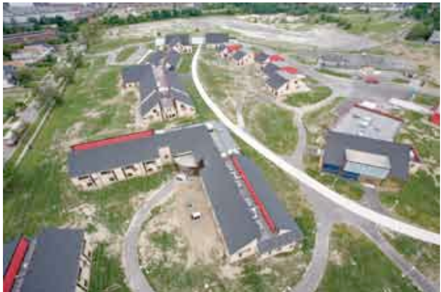
MOVING UP The 24-acre educational campus, located at East 140th Street and Coit Road in Cleveland's Collinwood neighborhood, includes nine buildings.
