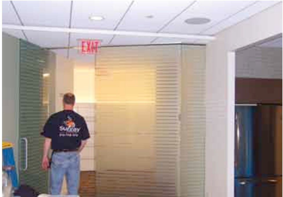
DESIGN DIFFERENCE Fasara decorative window films provide an etched appearance that is opaque and yet lets in light. When used in cubicles and in offices where there are inside windows and people walking by, etched glass lessens the distraction, because the window is opaque.
