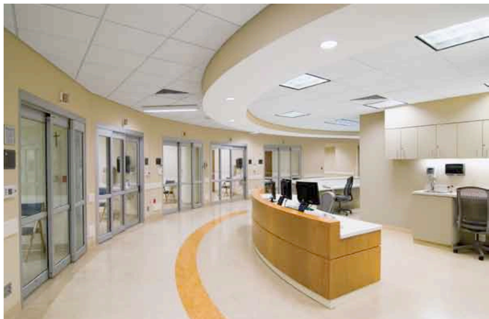
EASY ACCESS Glass bi-fold doors and single swing doors allow clear views and versatile access to patients.
