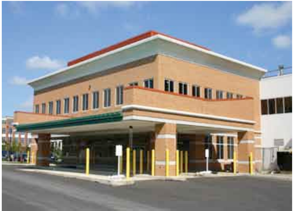
EASY MONEY A standing-seam metal roof is used on the three-bay drive-through canopy for tenant Huntington Bank.
