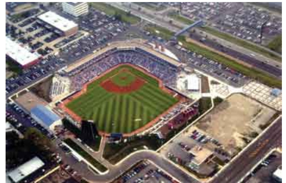
HITTING HOME CT Consultants has provided engineering services for many local projects, such as the Eastlake Ballpark, home of the Cleveland Indians Class A affiliate Lake County Captains.
