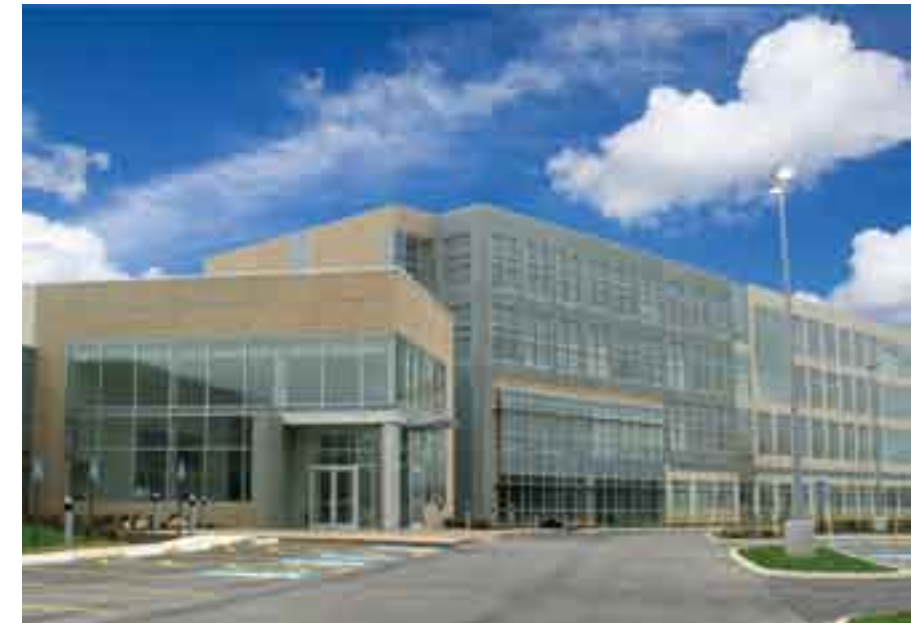
BUILDING BUSINESS The Cleveland-Cuyahoga County Port Authority has provided bond financing for various partners, including $6 million to Avery Dennison in September 2005.
