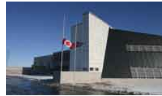
TWO FOR ONE Black metal paneling at the Toronto Pearson International Airport's Fire and Emergency Training Institute provide solar air heating while serving as a notable design feature.
