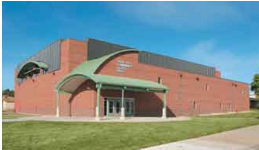
MONEY TALKS Community centers in Rapid City, South Dakota utilize solar air heating panels, providing ongoing cost savings while taking advantage of government tax credits.
