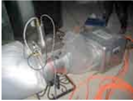
TIGHT WRAP Karpinski sealed supply ducts in the museum's original 1916 building.
