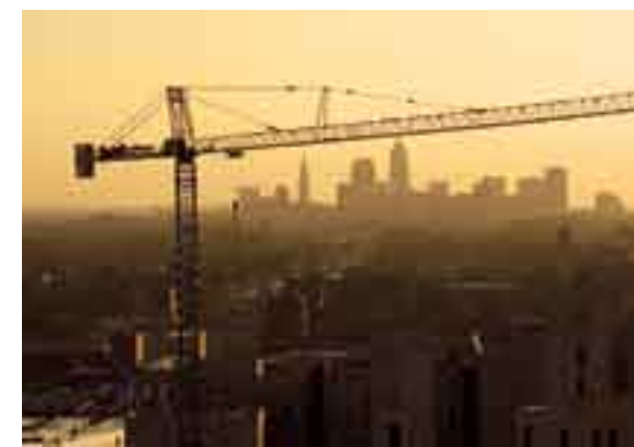
STILL ON THE SKYLINE "We started in Cleveland; we're here to stay," says ALL Erection & Crane Rental Sales Manager Norm Rados says.
