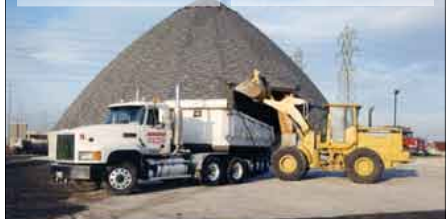
First Privately Owned Salt Dome Between Cleveland and the Atlantic Seaboard!
