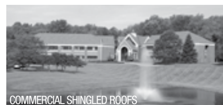
COMMERCIAL SHINGLED ROOFS
