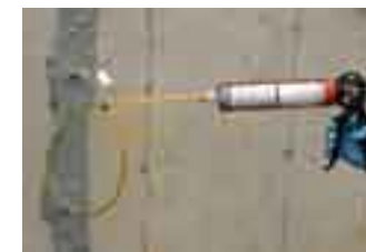
Emecole crack injection repair
