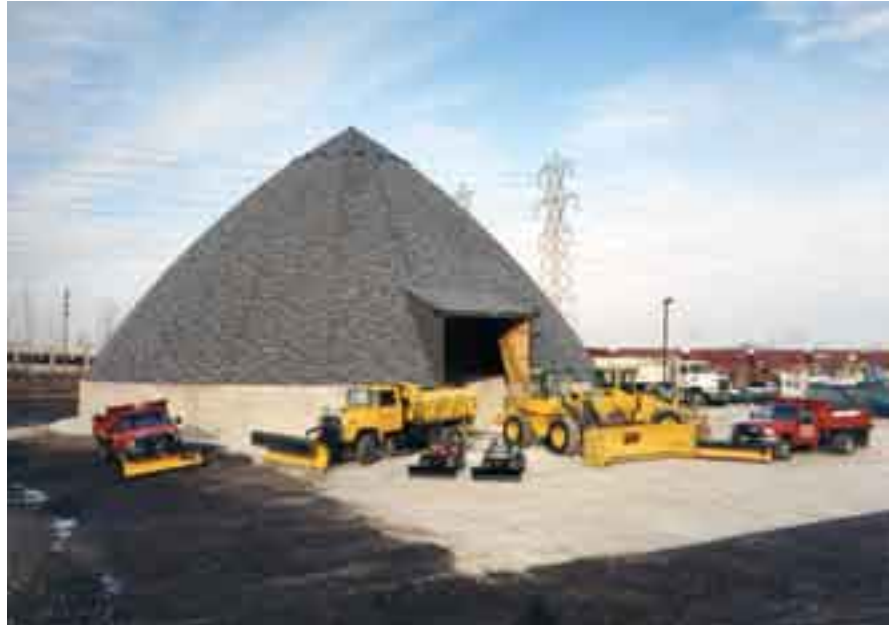
DRY DOME The Abraxus salt storage facility, located in Brooklyn, Ohio and open 24/7, is the first privately owned dome of its kind from greater Cleveland to the Atlantic seaboard.
