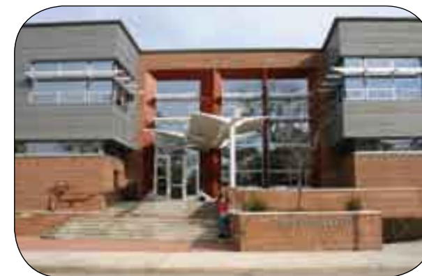
Proud to be part of the team that completed the Cleveland Heights - University Heights Public Library
