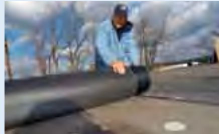
Installing Factory-Applied Tape
