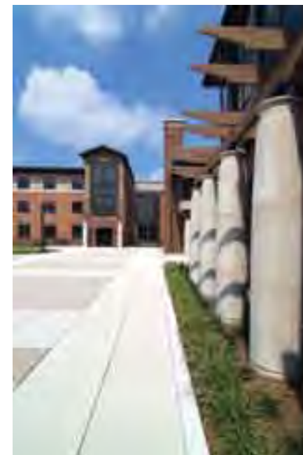
SUPPORTING HISTORY Concrete columns allude to the classical architecture of some buildings on the university's front campus.
