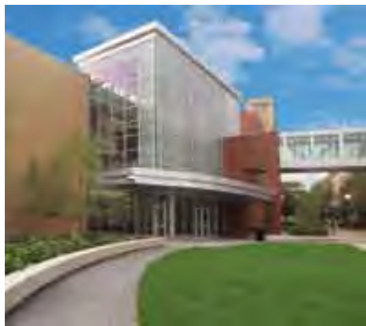
BRIGHT IDEA Energy savings at the recreation center are assisted by the use of ample daylight through glass exterior walls.
