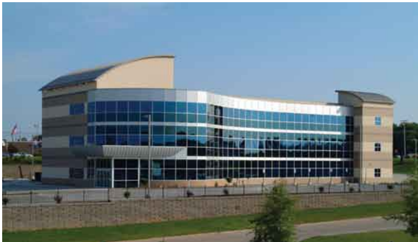
FLOOR BY FLOOR Originally designed as two stories, the concrete and brick ribbon-glassed structure was expanded to three, with the first floor housing the center and the two upper floors planned as medical offices for entities doing business with EMH.
