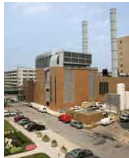
POWER PLACE The building houses new central chilled water equipment, emergency power generation and electrical distribution equipment.
