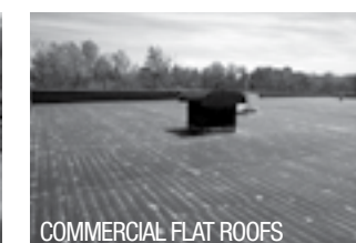
COMMERCIAL FLAT ROOFS
