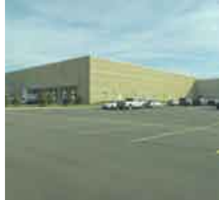
ROOM TO GROW A 900-space parking lot accounts for approximately 700 employees working at the facility, plus room for a growth capacity of 15-20%
