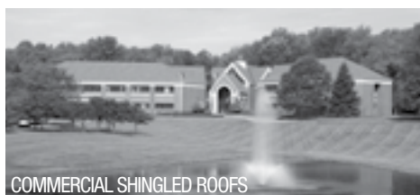
COMMERCIAL SHINGLED ROOFS
