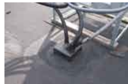
GOB STOPPER A roofer "flashed" a refrigerant line penetration at this site (left), yet could have installed a longer-lasting system (right).
