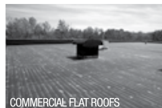
COMMERCIAL FLAT ROOFS
