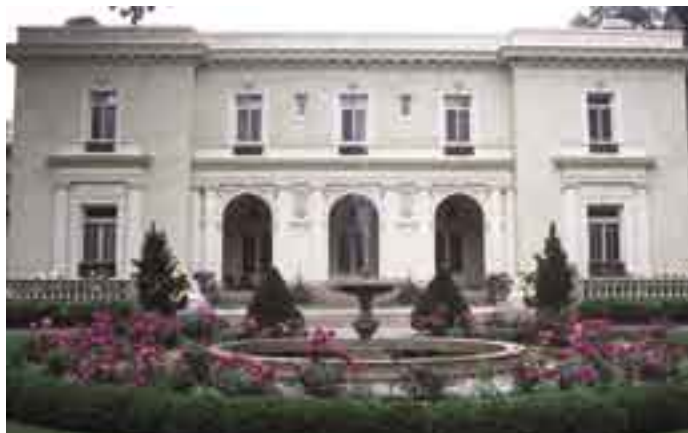
WATER WORKS A fountain, surrounded by roses and a boxwood hedge, has been added to emphasize the symmetry and elegance of the architecture. Balustrades surrounding the side terraces are also visible, with azaleas in front to soften the line and add color in spring.
