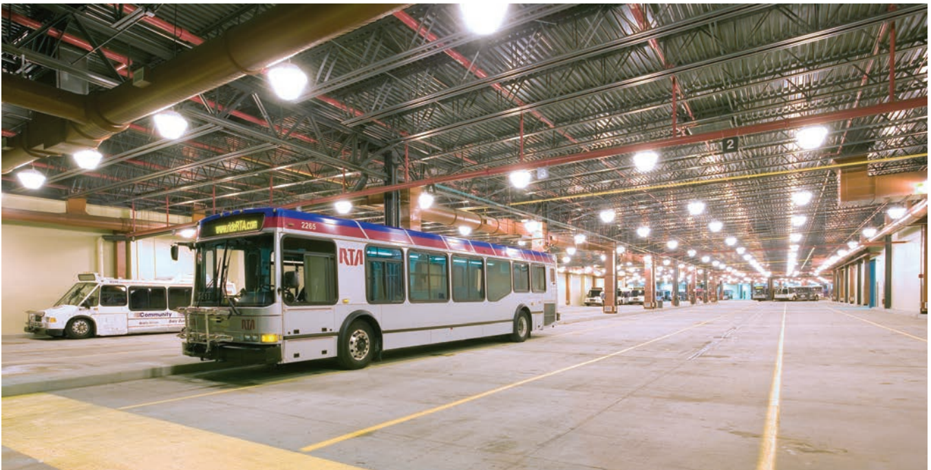
FINDING A FLOW Within the bus storage area, piping along the ceiling is color-coded according to system. Sloped floors in the garage guide water and other fluids into an industrial waste piping system.
