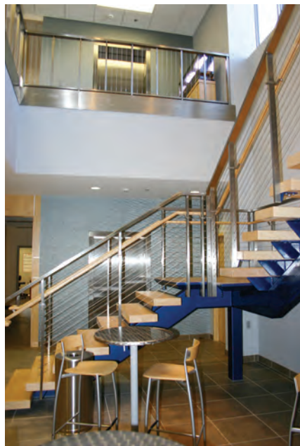
MOVING UP The stairwell, which is the building's centerpiece, required a major tear out of the existing second floor.
