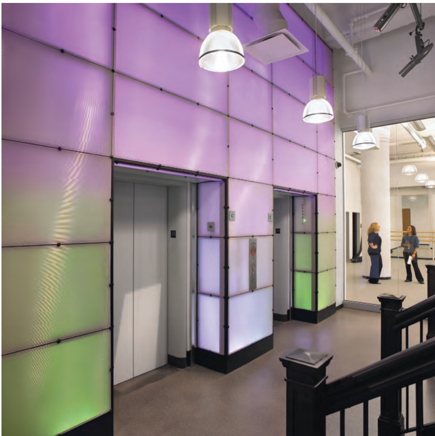
LIT UP The elevator lobby features a translucent plastic scrim lit from behind by LED light generators. The ColorBlast™ wall slowly changes color every few minutes.
