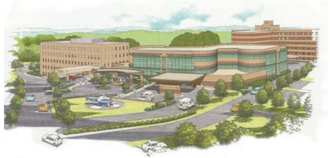
Renovated and expanded Marymount Hospital
