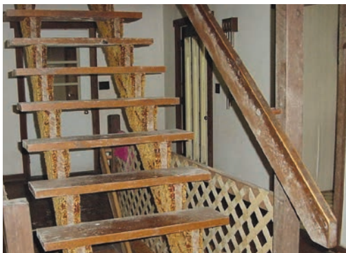
Typical view of interior mold
