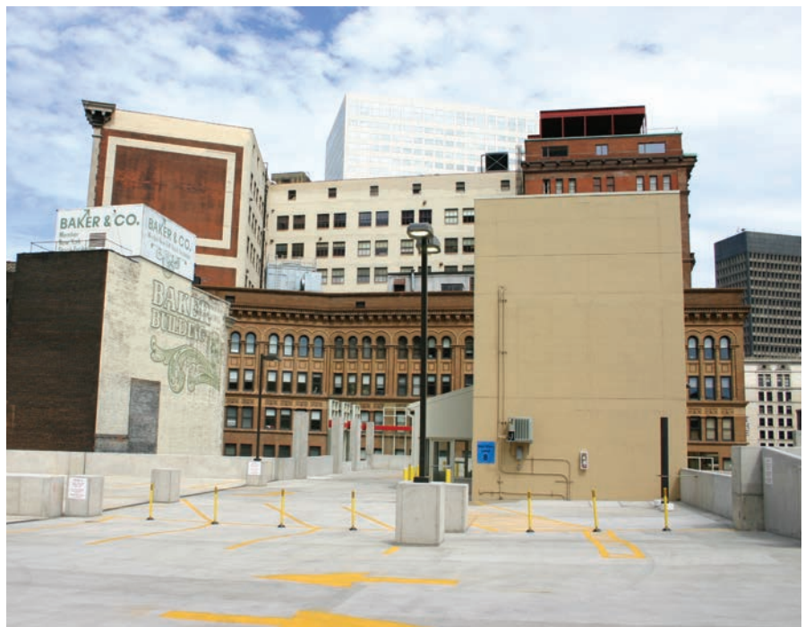
TOP TO BOTTOM This is the view from atop the 515 Euclid Avenue facility. It will actually start the bottom level of the 19-story condominium complex.
