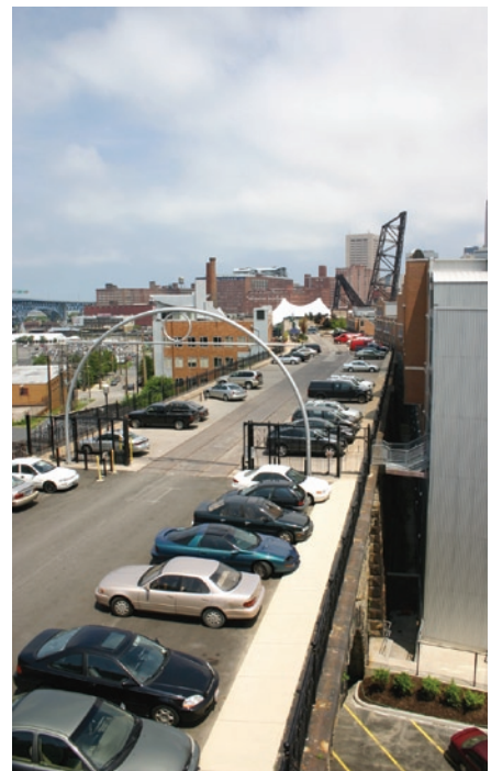
PULSE OF THE PROJECT The historic Detroit-Superior Viaduct is the integral centerpiece of the Stonebridge Development.
