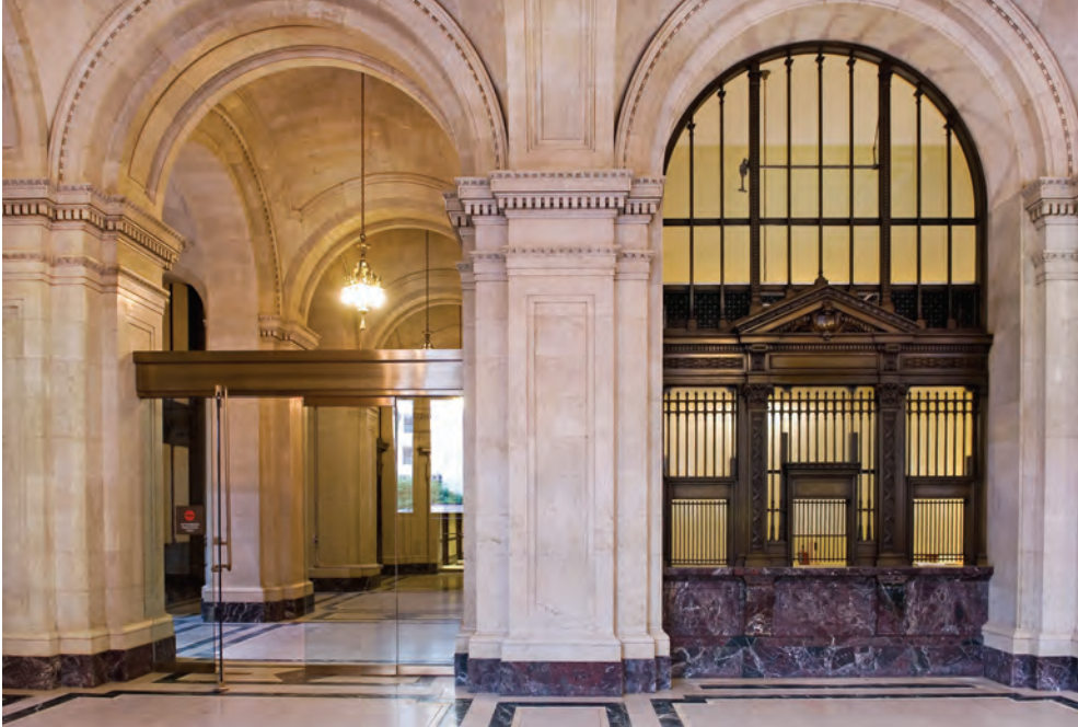
TOP TO BOTTOM The corridors, with stone floors, marble walls, plaster ceilings and mahogany doors and frames, required extensive refurbishment.
