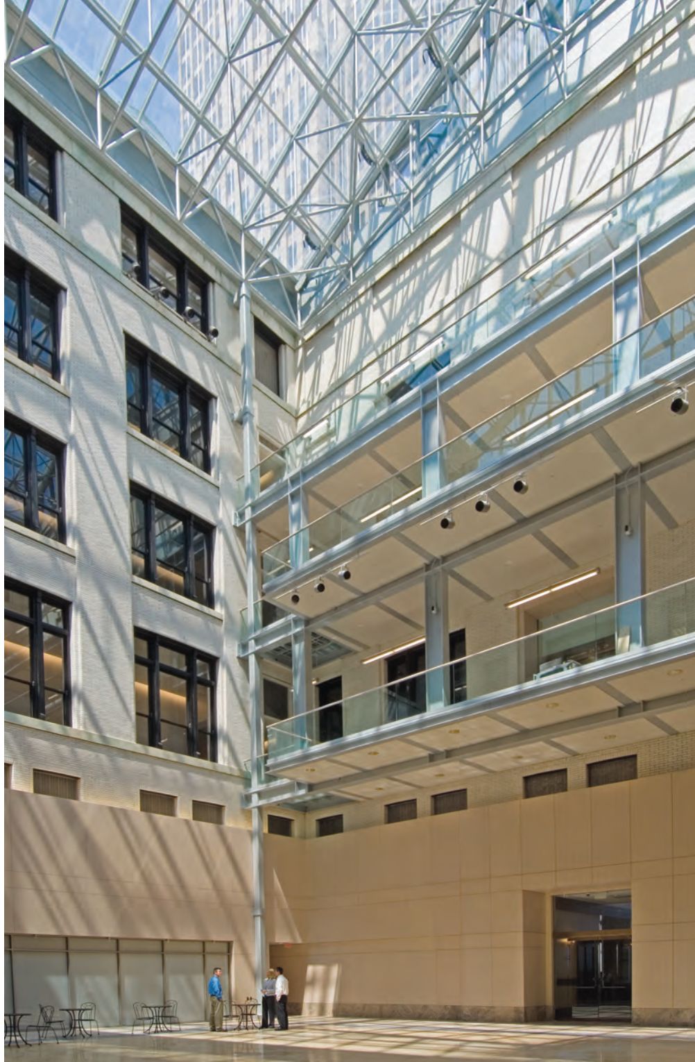
SEPARATE FOR SECURITY A former light court was converted to functional public space. Now, tenants and the public do not cross paths, which addresses a security concern.
