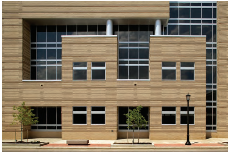
POWERFUL PATTERN Viewed from a distance, the rows of windows on every floor form a vertical pattern against the exterior Berea Sandstone™.
