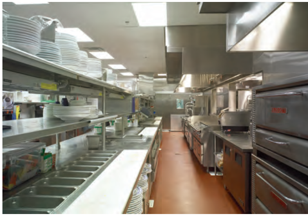
SOME LIKE IT HOT In the club's kitchen, a polyurethane-coated floor offers thermal-shock protection.
