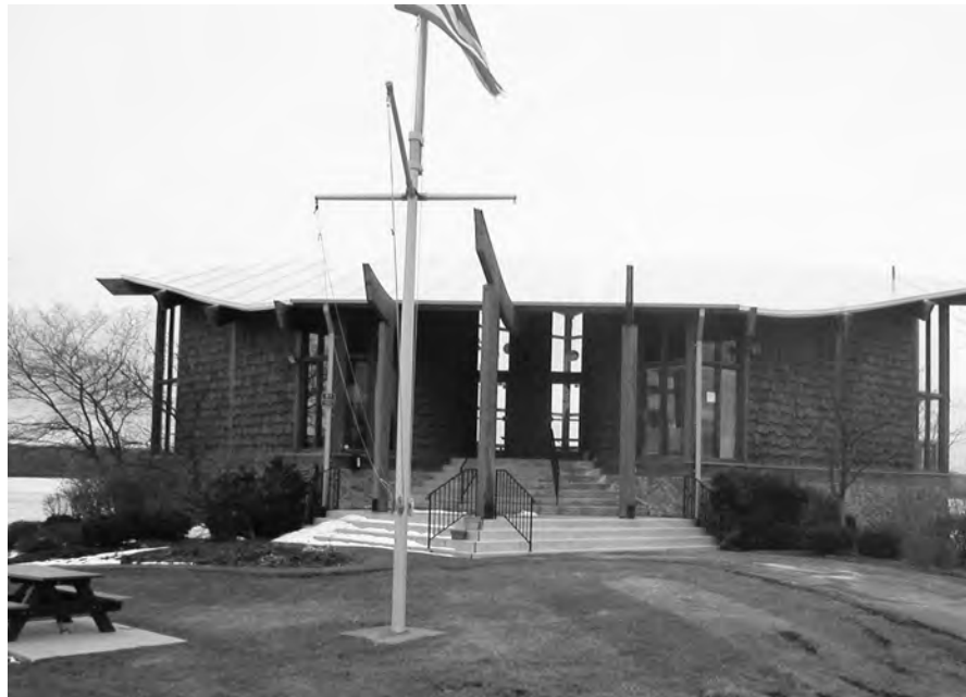
SMALL PROJECT, CONSIDERABLE CHALLENGES During Preferred Roofing's work at the marina community center, special care had to be taken in the planning process as the fasteners were not permitted to penetrate through the decking into the marina's interior.
