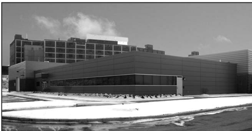
F.B.I. Automotive & Electronic Communication Processing Facility
