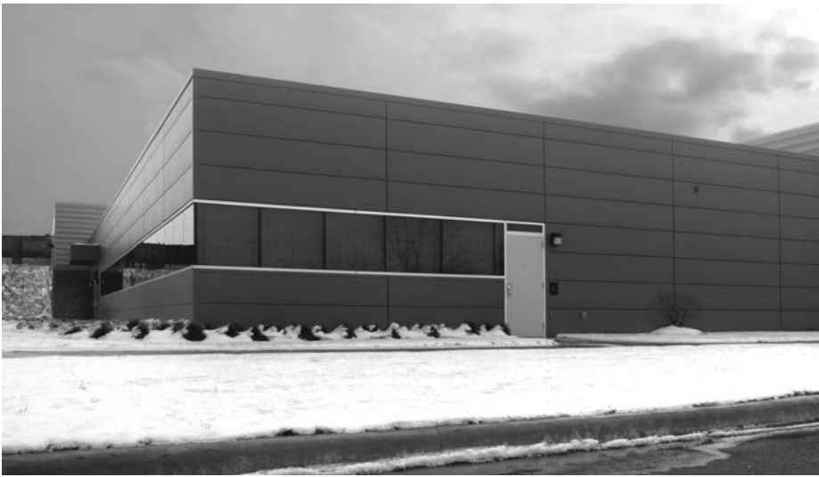
Metal panels with a window ribbon comprise the office exterior.
