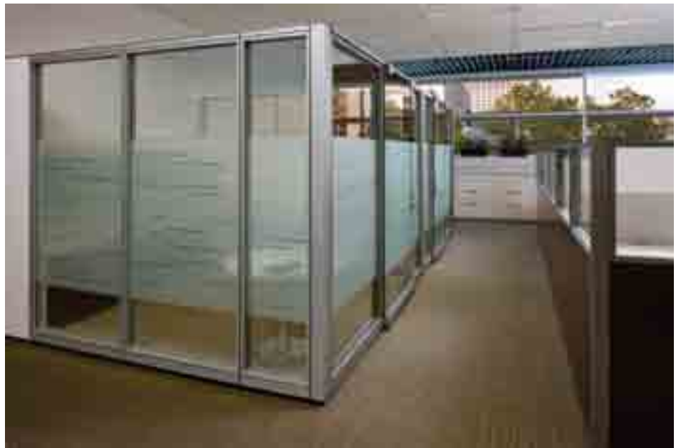
SECURED STYLE Throughout the facility, the design team used various glass films to control visual privacy in certain areas.
