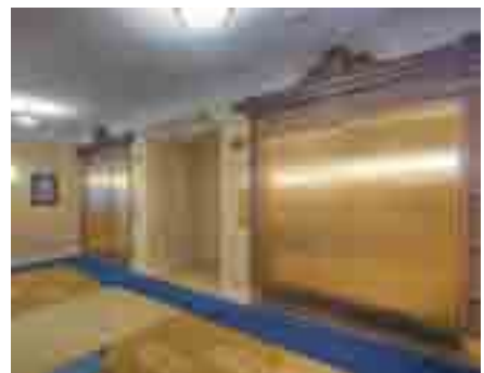
PAINSTAKING PRESERVATION The elevator frame in the lobby was restored to its original brass, a process which included removing nearly 80 coats of paint.
