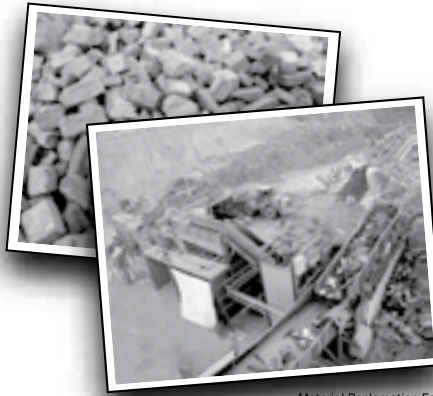
Material Reclamation Facility
