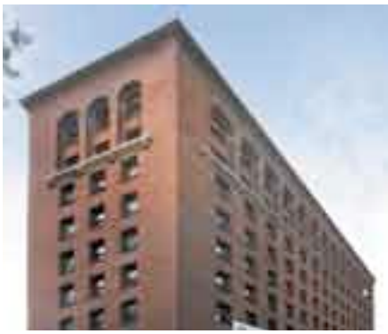
PIECE OF THE PAST Built in 1927, the Meritus House Building was designed by famed Cleveland architectural firm Hubbell and Benes Company.
