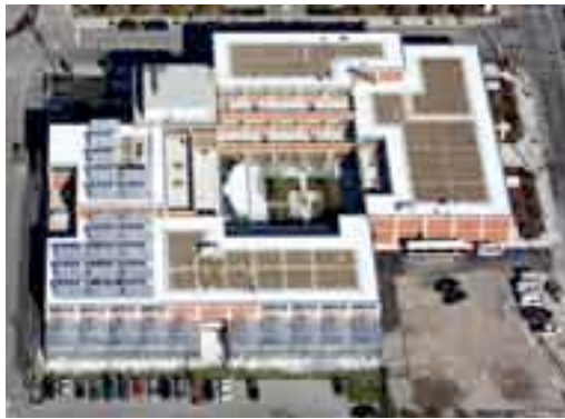
GREEN TO GO Solon-based W. P. Hickman Systems, Inc. supplied a key feature at Chicago's Pacific Garden Mission: a green roofing system incorporating a solar-reflective membrane and vegetative grids.
