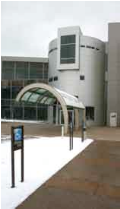
COMING AROUND A cantilevered arc, glass canopy (left) has been added to the original entrance at Parker's headquarters. Inside the entrance lobby (right), the company's global presence is represented by a series of five suspended, illustrated scrimms.
