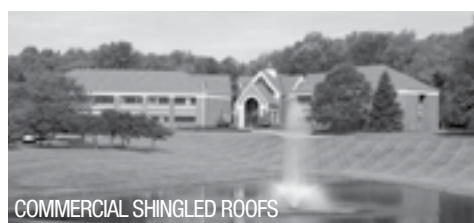
COMMERCIAL SHINGLED ROOFS
