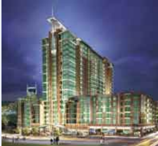
GOING UP, DOWN SOUTH Cleveland's ka Architecture designed ICON in the Gulch, a mixed-use development currently under construction in Nashville
