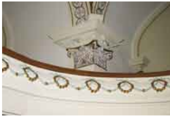
SHINE ON New HID lighting was installed to illuminate columns in the church.
