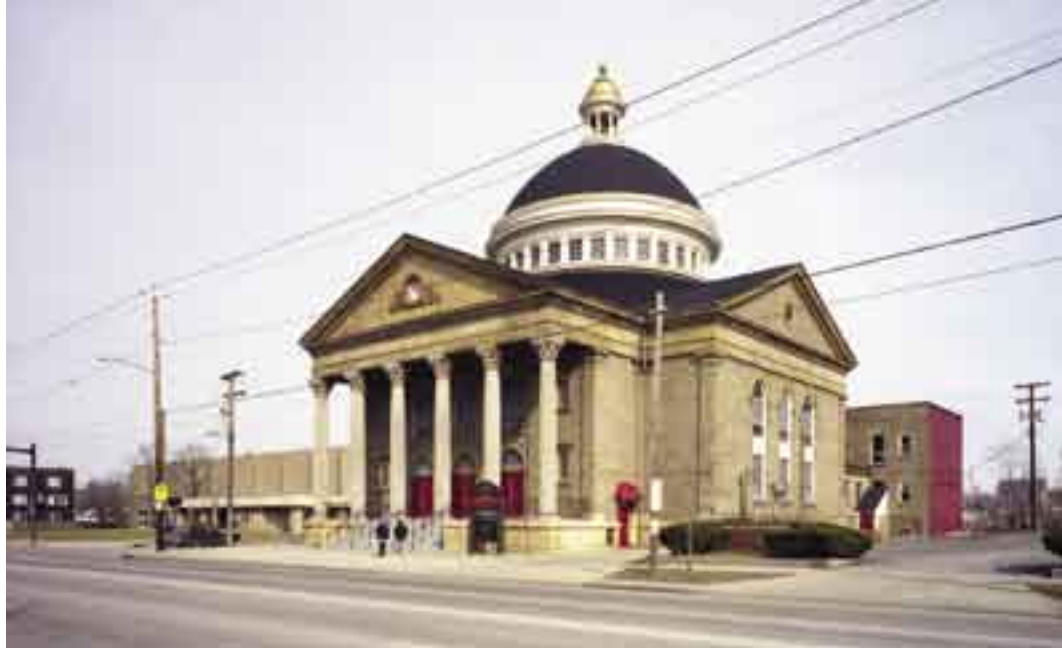
FIRST LOOK The initial phase of the project included buttoning up the outside of the building in order to make the church watertight.
