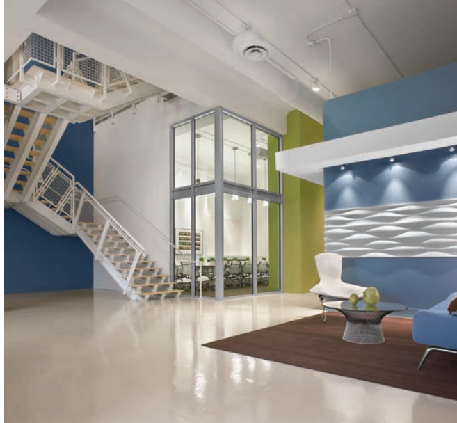
DOWN TO BUSINESS A steel-framed, rectangular stairwell with bamboo treads and multiple levels was constructed in the lobby of Vocon's new headquarters.
