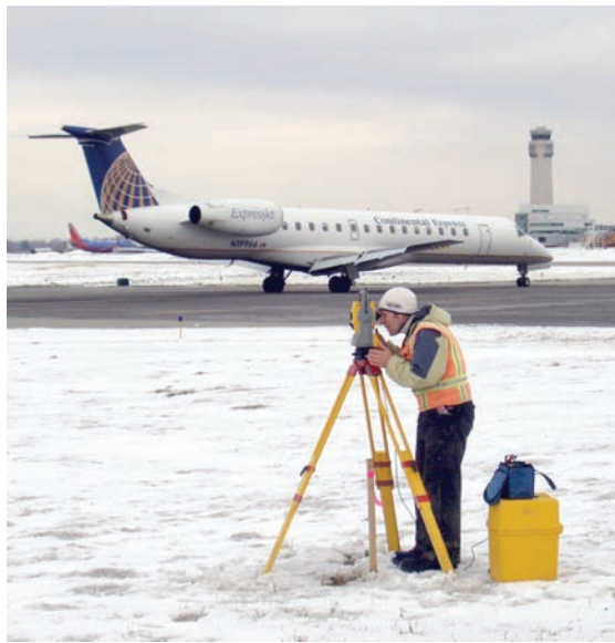
WIDE LOOK KS Associates operates one of Northern Ohio's largest surveying groups, providing services such as topographic, boundary and utility location surveys.
