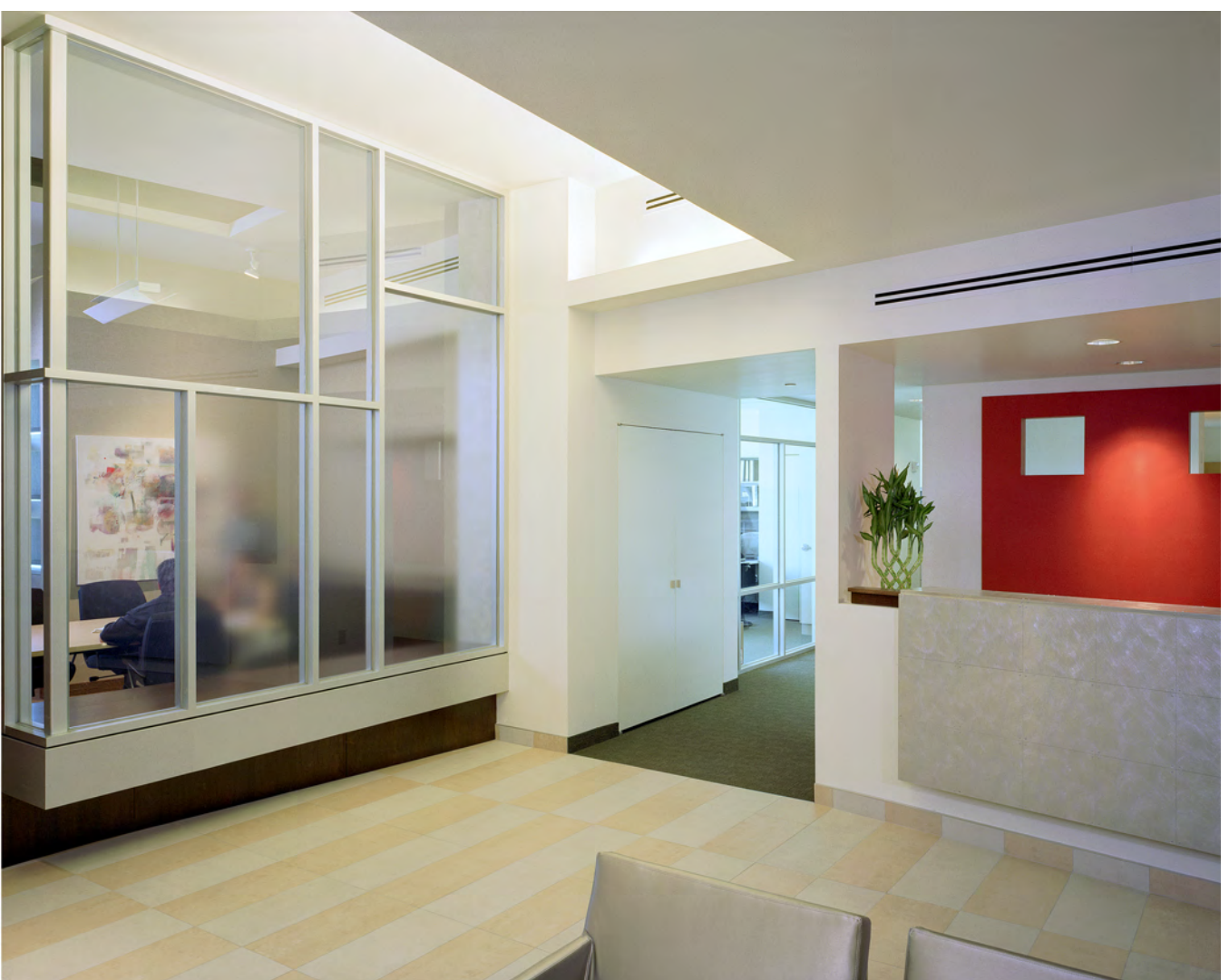
CLEAR CHOICES Framed glass walls can be found throughout, beginning with one separating the reception area from the elevator lobby. This glass structure demonstrates versatility with sections of varying clarity; some textures are clear while others are blurry.
