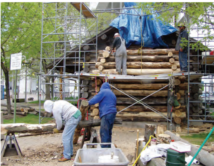
WOOD WORK Power tools were used during the restoration, as were older tools including drawknives to pull bark away from logs.
